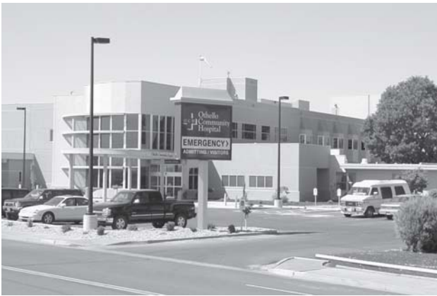
Othello Community Hospital addition
